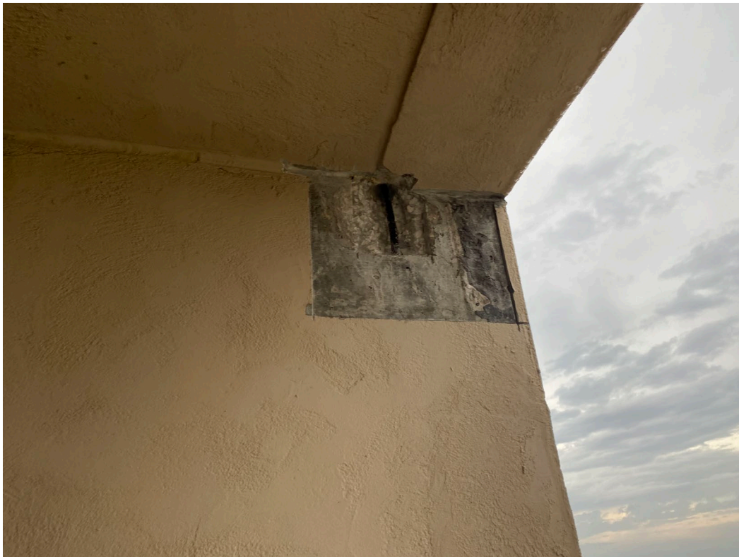
Picture 2: Typical wall excavation
