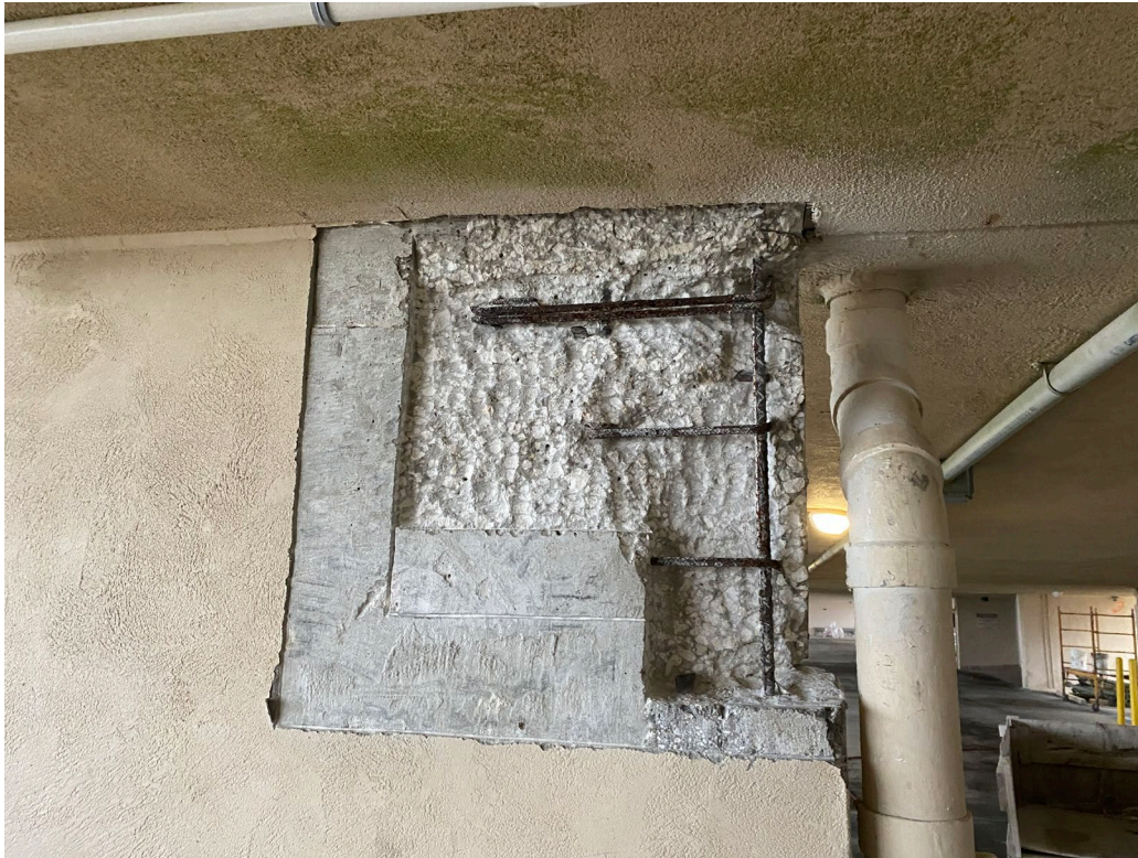
Picture 3: Typical wall excavation
