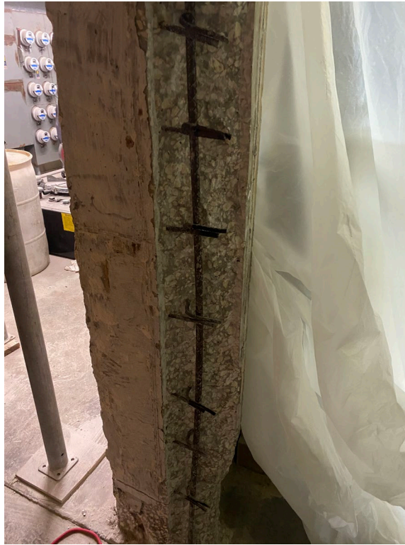
Picture 1: Wall excavation at the maintenance room door
